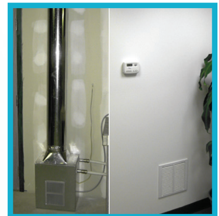
Behind wall Finished Room
